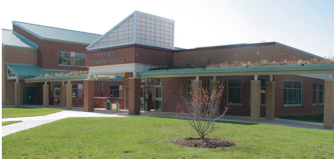
SCHOOL ENTRANCE SHOWING AWNING WITH GREEN ROOF CANOPY ON THE SIDEWALK
