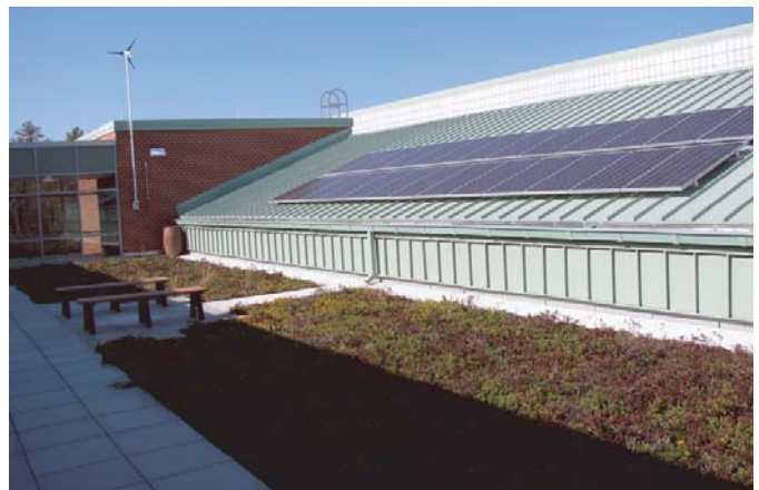
GREEN ROOF LEARNING LAB WITH SOLAR PANELS
