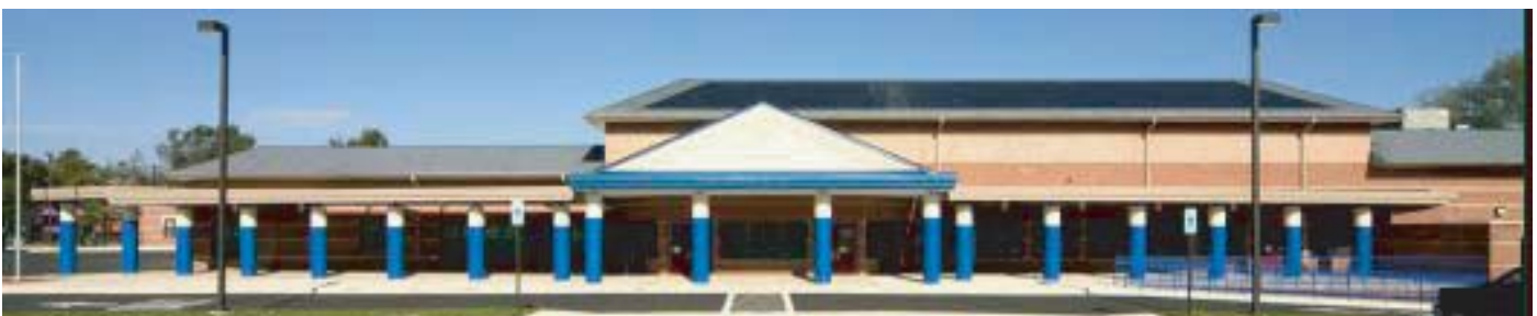
NEW ENTRY TO SCHOOL WITH PHOTOVOLTAIC (PV) SHINGLE ARRAY ON
