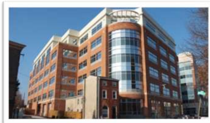
Whiting-Turner. UMD BioPark Building II
